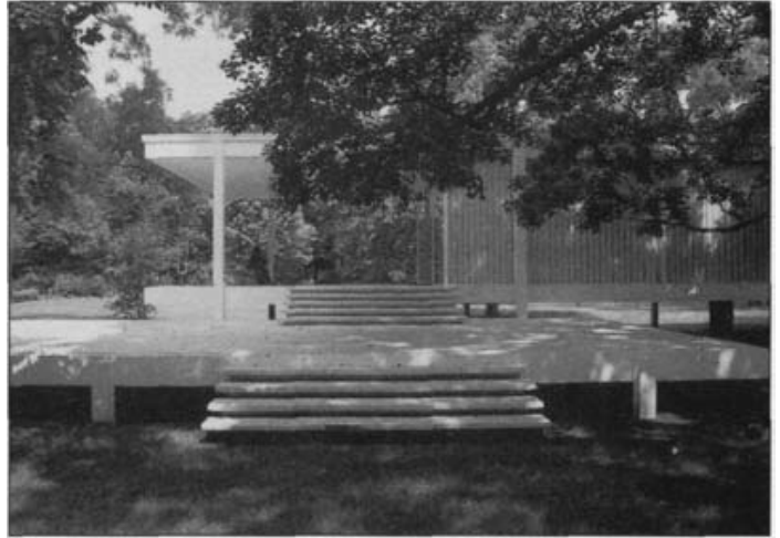
Fig. 3.8 The Farnsworth House, Illinois, USA, 1951. Ludwig Mies van der Rohe, architect. The mass-produced structural steel beam and column I-sections form important elements in the aesthetic vocabulary of this building.
