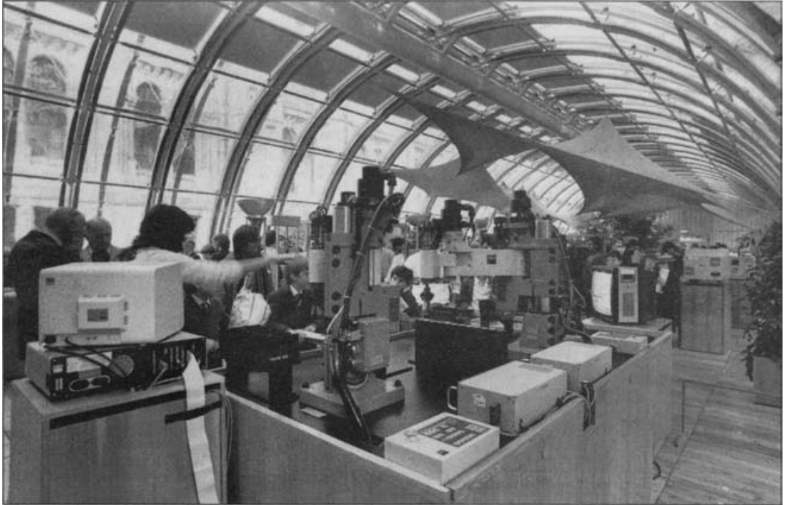
Fig. 1.12 Building for IBM Europe travelling exhibition. Renzo Piano, architect/engineer, Ove Arup and Partners, structural engineers. A complex, highly efficient vaulted structure like this would not normally be used for a short-span enclosure. It was justified in this case due to a requirement for a lightweight structure for a portable building. The choice of lightweight materials - timber and plastic-was also sensible. [Photo: Ove Arup & Partners]
