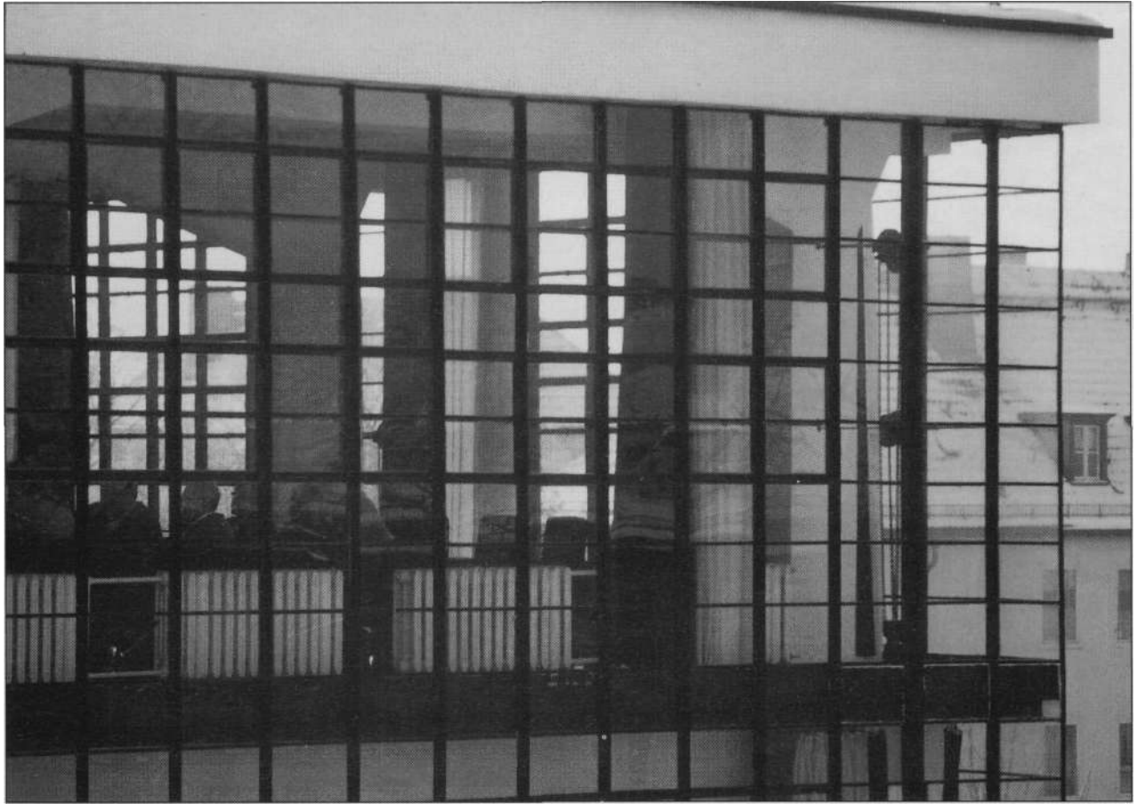
Fig. 4.7 The Bauhaus, Dessau, 1926, Walter Gropius, principal architect. This building had a reinforced concrete frame structure which provided the same opportunities for new architectural expression as had been recognised by Le Corbusier. The glazed curtain wall which rises through the upper floors of the building represents an exploitation of one of those opportunities. [Photo: Paul H. Gleye]
