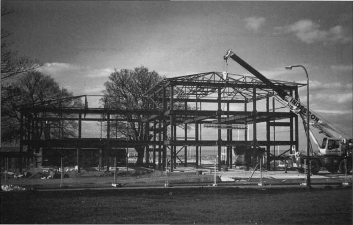
Fig. 1.15 The high strength of steel allows the creation of structures with very slender elements. In buildings which are supported by steel frameworks the volume occupied by the structure is low in relation to the total volume of the building. (Photo: A. Macdonald).
