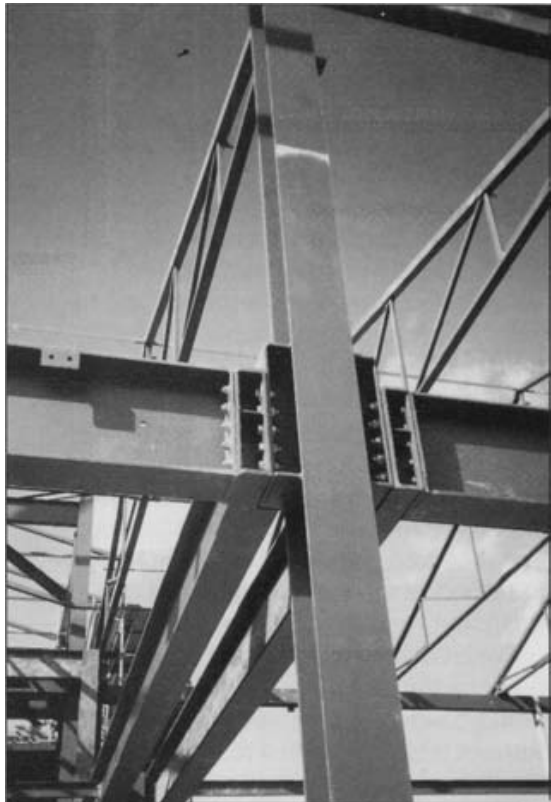
Fig. 1.15 The high strength of steel allows the creation of structures with very slender elements. In buildings which are supported by steel frameworks the volume occupied by the structure is low in relation to the total volume of the building. (Photo: A. Macdonald).
