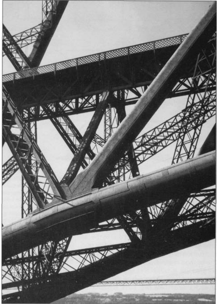
Fig. 1.23 Forth Railway Bridge, Scotland, 1882-90, Henry Fowler and Benjamin Baker, engineers. The railway track is carried on an internal viaduct which is supported at the junctions of the triangulated main structure. [Photo: A. Macdonald]
