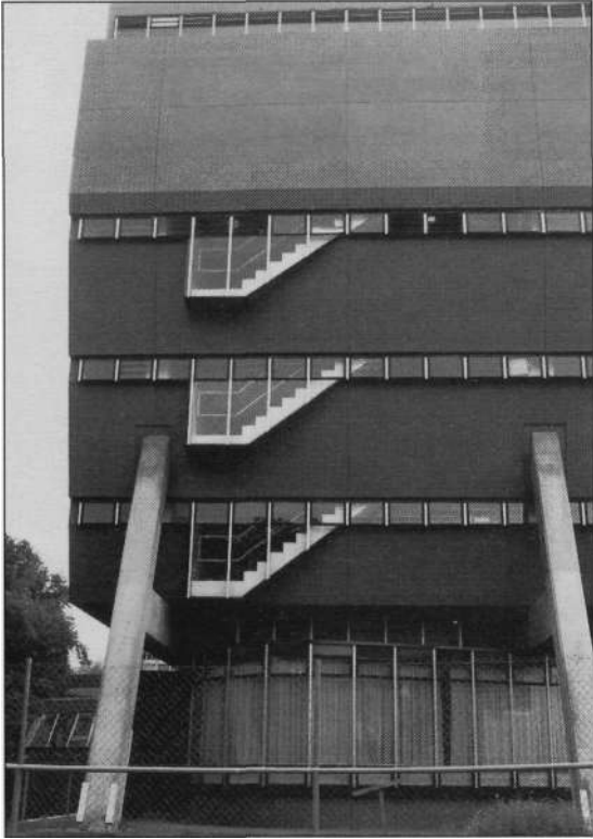
Fig. 4.16 Florey Building, Oxford, England, 1971. James Stirling, architect, F.J.Samuely & Partners, structural engineers. The stairs which protrude from the inwardly canted rear wall of the Florey Building provide a good illustration of the type of complexity which the mouldability and structural continuity of a reinforced concrete structure allow (Photo: P. Macdonald).
