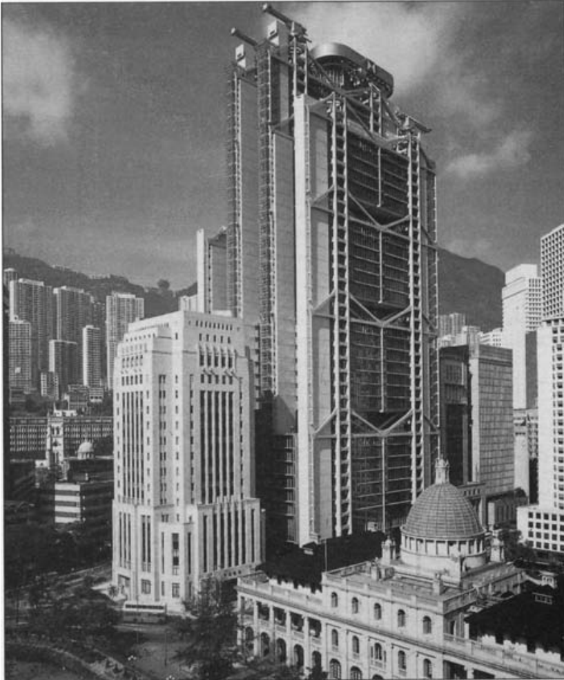
Fig. 1.3 HongkongBank Headquarters, Hong Kong, 1979-84. Foster Associates, architects. The structure of this building is expressed prominently both on the exterior and in the interior. It contributes directly as well as indirectly to the appearance of the building. [Photo: Ian Lambot. Copyright: Foster & Partners]
