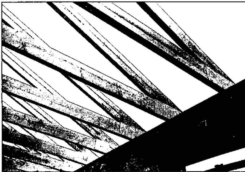
Fig. 6.38 Punched-metal-plate fasteners, which form combined nail-and-gusset plate units, are used as the fastening elements in these trussed rafters.
