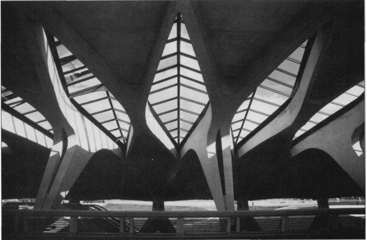
Fig. 1.11 TGV Station, Lyon-Satolas, France 1989-94, Santiago Calatrava, architect/engineer. A vaulted structure in reinforced concrete is used here to achieve a relatively long span. [Photo: E. & F. McLachlan]
