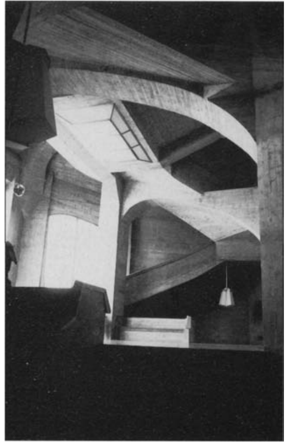
Fig. 1.17 Goetheanum, Eurhythmeum, 'Glashauss' studio, Dornach, Switzerland, 1924-28. Rudolf Steiner, architect. The complexity of form which is possible with in situ reinforced concrete is well illustrated here. [Photo: E. & F. McLachlan]
