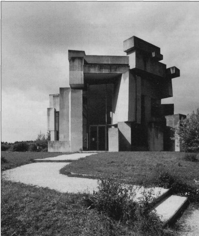
Fig. 4.1 Church, Vienna, Austria, 1965-76. Fritz Wotruba with Fritz G. Mayr, architects. The expressive possibilities of reinforced concrete are well illustrated here. [Photo: E. & F. McLachlan]
