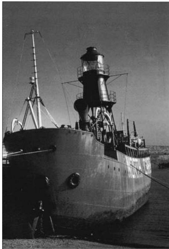
Fig. 2.3 Steel can be fabricated into almost any shape as the structures which are built for the marine environment demonstrate. The construction of a ship requires techniques of fabrication which are significantly more complex and expensive than those which are normally used in the construction of buildings. There is, nevertheless, no technical reason why such shapes should not be employed in architecture. [Photo: P. Macdonald]
