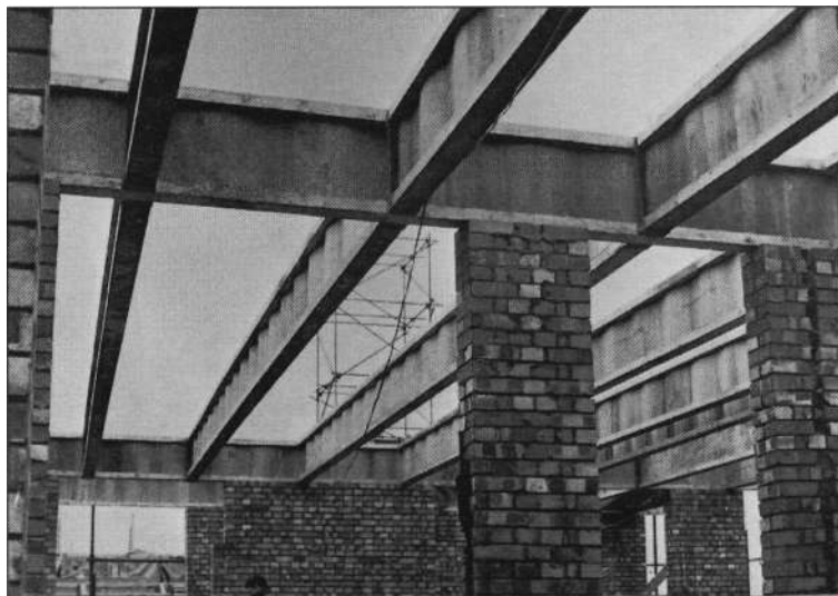
Fig. 6.41 Plyweb built-up-beams at close spacing are used here to form the principal structural elements of a roof deck. The arrangement is similar to that of a traditional joisted deck with sawn-timber elements. The use of built-up-beams allows longer spans to be achieved.
