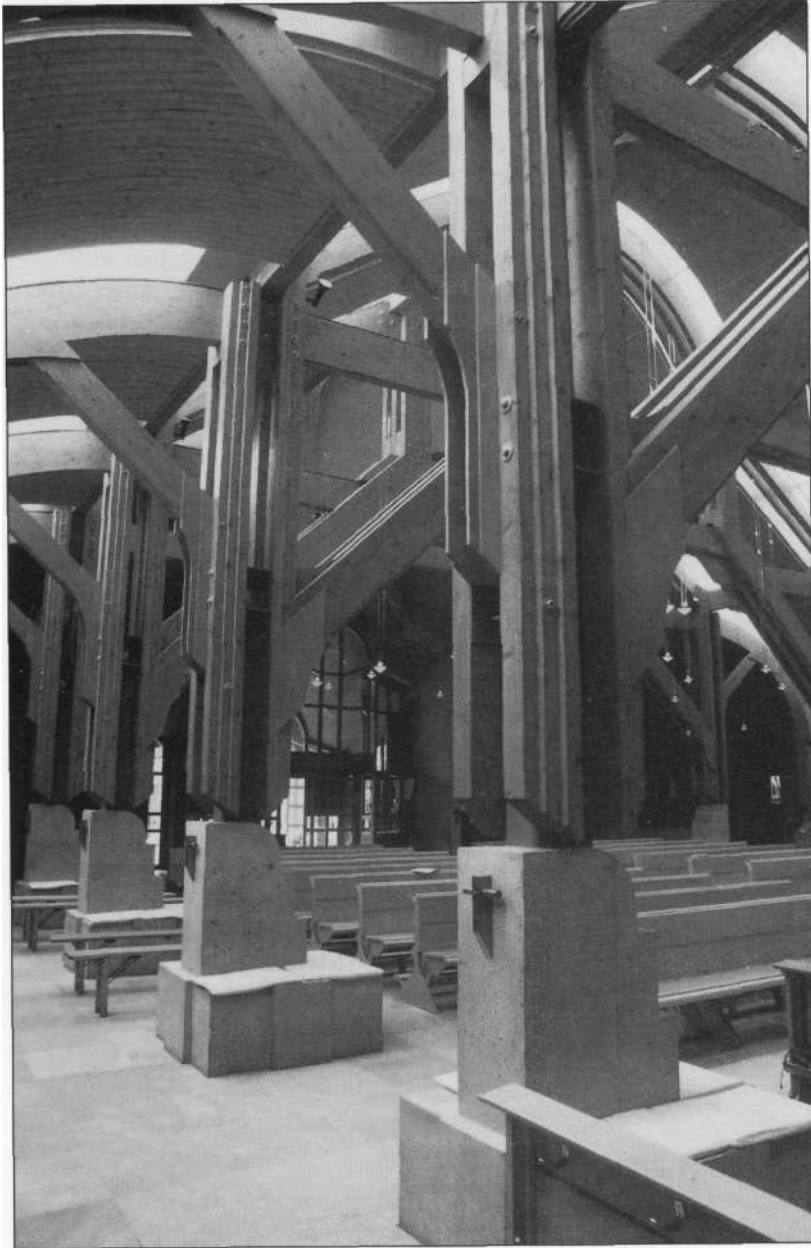
Fig. 6.15 Ragnitz Church Hall, Graz, Austria, Szyszkowitz and Kowalski, architects. The roof of this building is supported by a timber skeleton framework which has a significant architectural presence. [Photo: E. & F. McLachlan]
