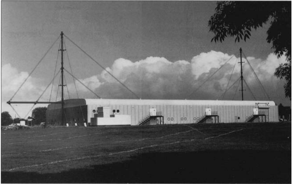
Fig. 3.44 Ice Rink, Oxford, 1984. Nicholas Grimshaw & Partners, architects; Ove Arup & Partners, structural engineers. The mast-and-tie system was used here to achieve a large column-free interior. The prevailing ground conditions were a factor in the selection of this particular structural configuration. [Photo: Ove Arup & Partners]
