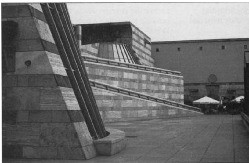
Fig. 1.4 Staatsgalerie, Stuttgart, Germany, 1980-83, James Stirling, architect. This building has a reinforced concrete structure and non-structural cladding. Although the structure plays a vital role in the creation of the complex overall form it is not a significant element in the visual vocabulary. [Photo: P. Macdonald]
