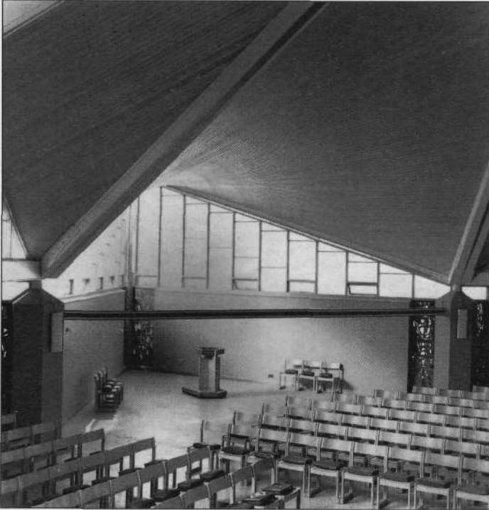
Fig. 6.59 Timber hyperbolic paraboloid shells are used here to form a roof structure of distinctive shape.
