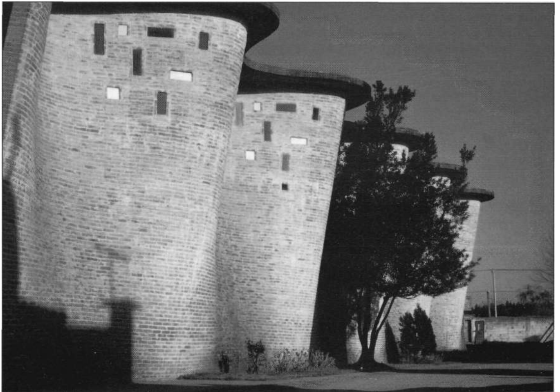
Fig. 5.8 Church at Atlantida, Uruguay, 1958. Eladio Dieste, architect. The plan-form of the walls of this building is that of a sinusoidal curve whose amplitude is greatest at the level where the bending moment is highest. The arrangement allows a large overall thickness of wall to be achieved with a minimal volume of masonry. This is a modern equivalent of the flying buttress. [Photo: Vicente del Amo]
