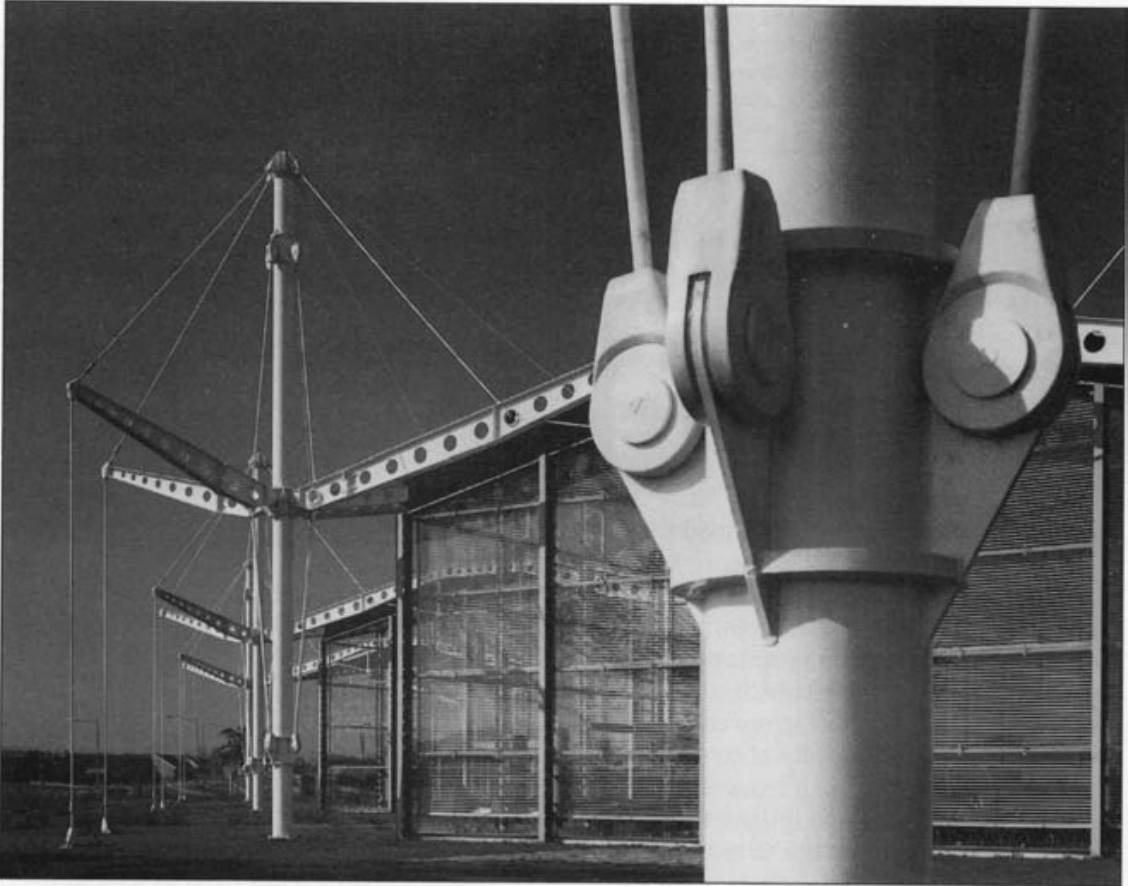
Fig. 3.14 Renault Sales Headquarters, Swindon, England, 1983. Foster Associates, architects; Ove Arup & Partners, structural engineers. Steel castings are used for the jointing components of complex shape which occur at the ends of the tie bars in this connection. [Photo: Alastair Hunter]
