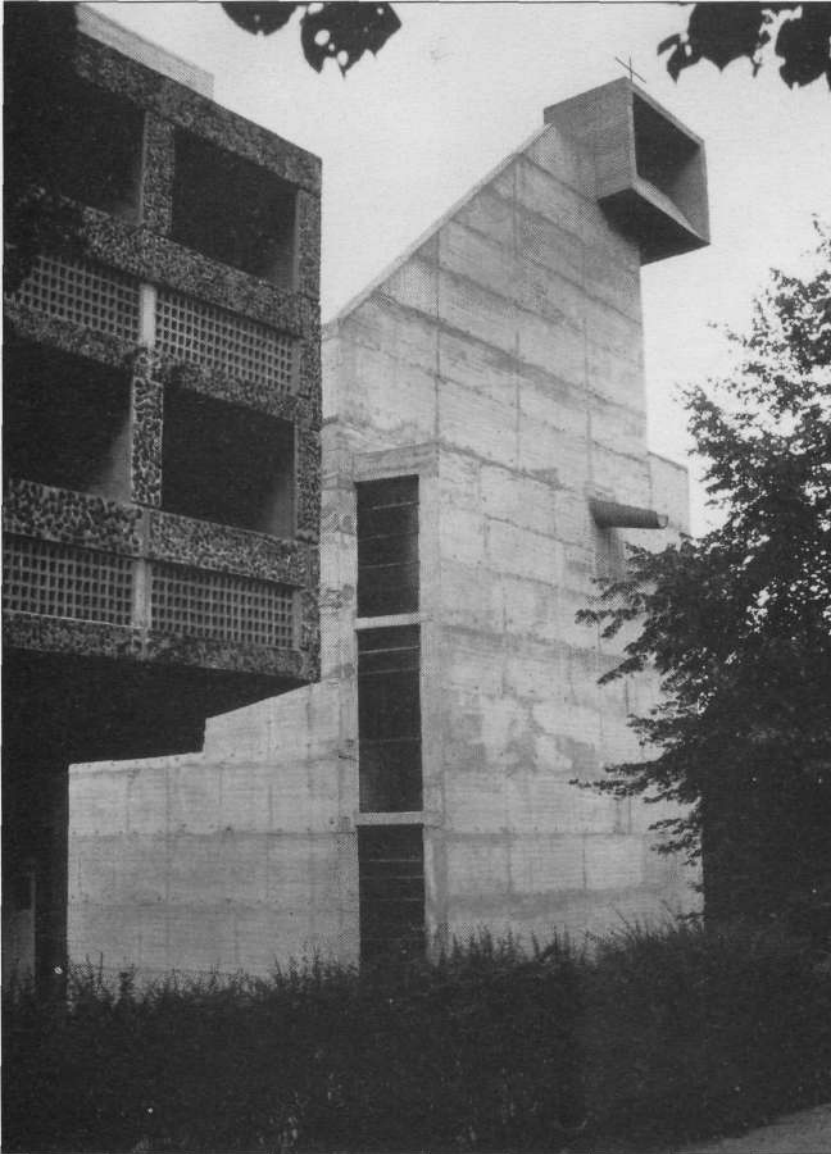
Fig. 4.10 Monastery of La Tourette, Eveux, France, 1955. Le Corbusier, architect. Exposed structural concrete, which bears the marks of the rough formwork against which it was cast, was a notable aspect of the architectural vocabulary employed by Le Corbusier in this period. It was compatible with his architectural thinking at that time but was also ideally suited to the requirements of this particular client and project. [Photo: Andrew Gilmour]
