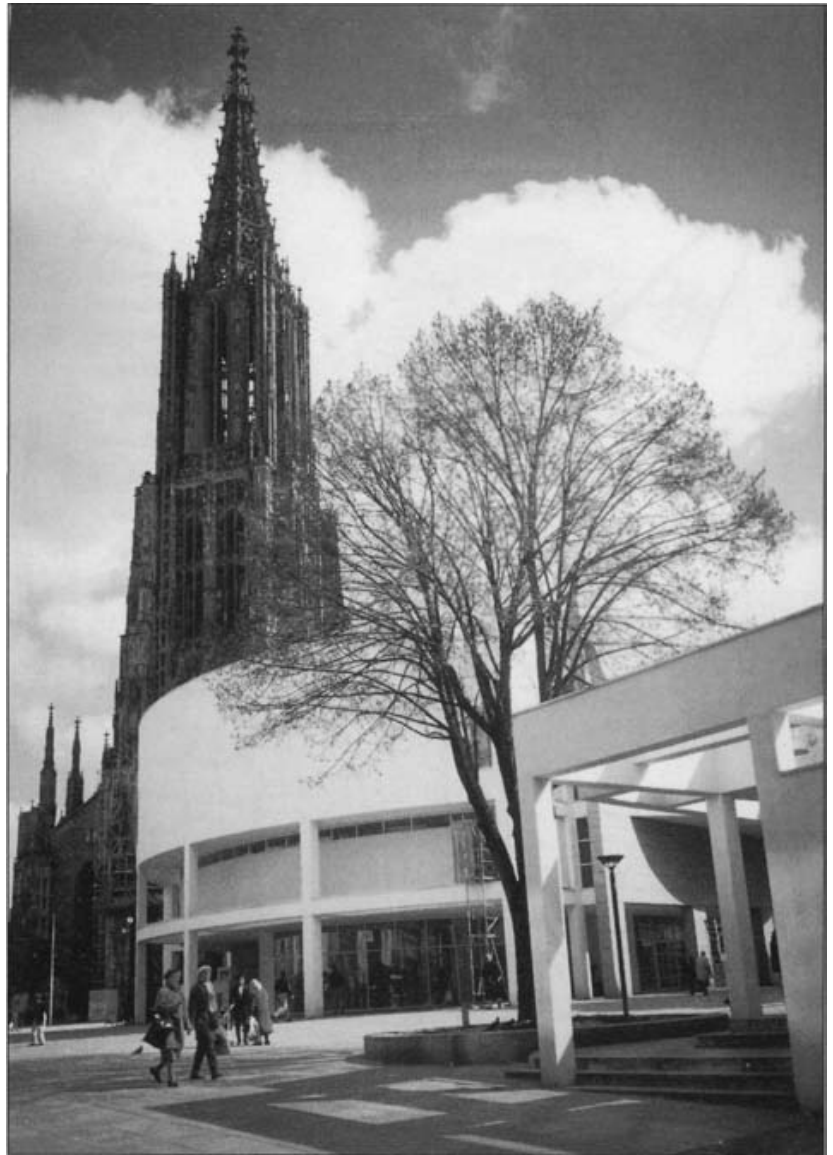
Fig. 2.13 Exhibition and Assembly Building, Ulm, Germany, 1993. Richard Meier, architect. The relatively complex form of this building was accommodated by a structure which was a relatively straightforward adaptation of one of the standard reinforced concrete arrangements. [Photo: E. & F. McLachlan]
