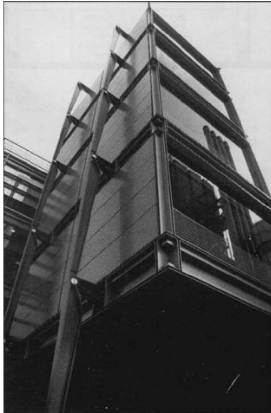
Fig. 3.1 Channel 4 Headquarters, London, England, 1994. Richard Rogers & Partners, architects. Concepts such as neatness, precision and high quality control are readily conveyed by the use of an exposed steel structure. [Photo: E. & F. McLachlan]
