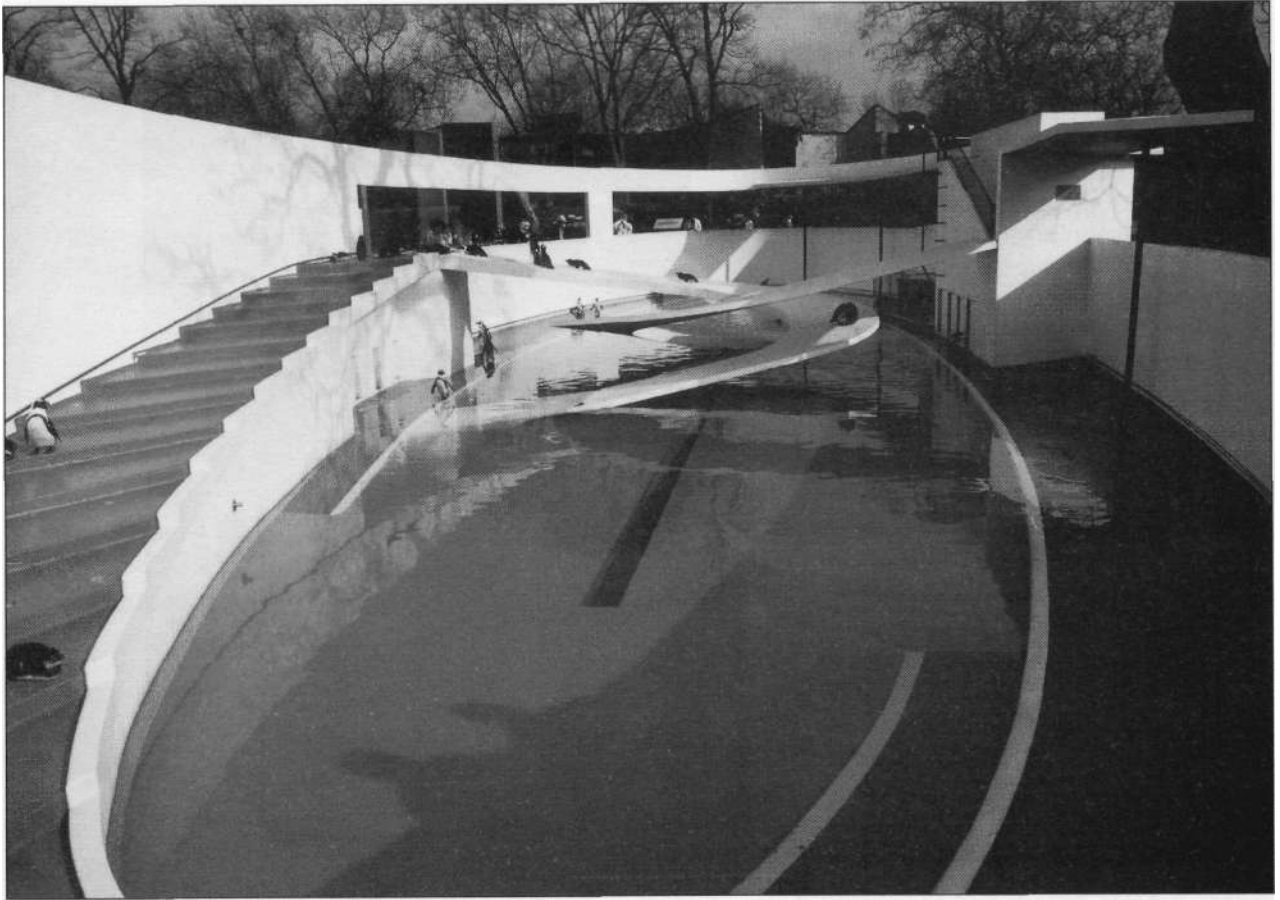
Fig. 4.9 Penguin Pool, London Zoo, London, England, 1933. Berthold Lubetkin and Tecton, architects; Ove Arup, structural engineer. The expressive possibilities of continuous structures of reinforced concrete are most eloquently demonstrated here. [Photo: E. & F. McLachlan]
