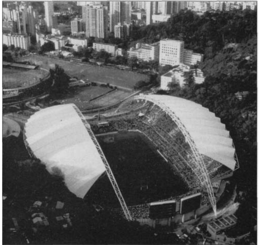
Fig. 3.10 Hong Kong Stadium, Hong Kong, 1995. Ove Arup & Partners, structural engineers. The principal structural elements of this long-span structure are steel arches which have a space-framework configuration. (Photo: Ove Arup Partnership)
