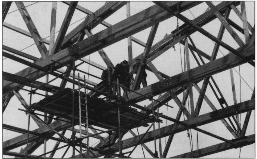
Fig. 6.33 Detail of large one-off timber truss.
