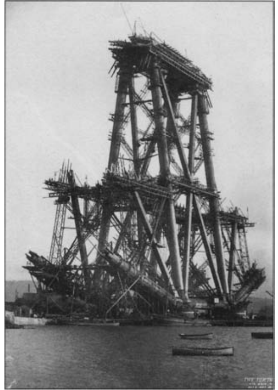
Fig. 1.21 Forth Railway Bridge, Scotland, 1882-90, Henry Fowler and Benjamin Baker, engineers. The main part of the structure consists of three pairs of balanced cantilevers. In this shot the central tower of one pair of cantilevers has been completed and the first elements of the cantilevers themselves have been added. The arrangement was adopted so that the uncompleted structure could be self-supporting throughout the entire period of construction. [Photo: E. Carey; copyright: British Rail Board Record Office]
