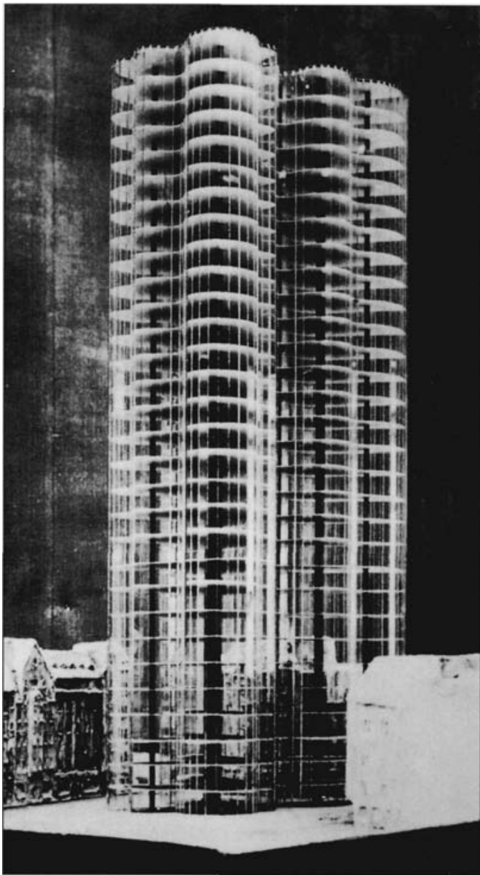
Fig. 3.4 Glass skyscraper project, 1922, model. Mies van der Rohe, architect. In the early twentieth century many visionary architects considered mass-produced high quality glass to be the ultimate modern building material, principally because it allowed the exterior of a building to be 'dematerialised'. The almost featureless high-rise structure faced in glass was an important architectural innovation of the early modern period.
