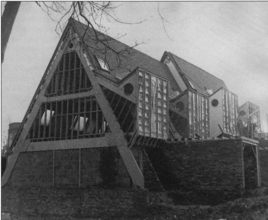
Fig. 6.1 Timber houses with skeleton-frame structures in which the principal elements are A-frames of plywood box-section. A characteristic of timber skeleton frameworks is that the primary structural elements are normally fairly large and must be incorporated into the aesthetic scheme of the building [Photo: Finnish Birch Plywood Association].
