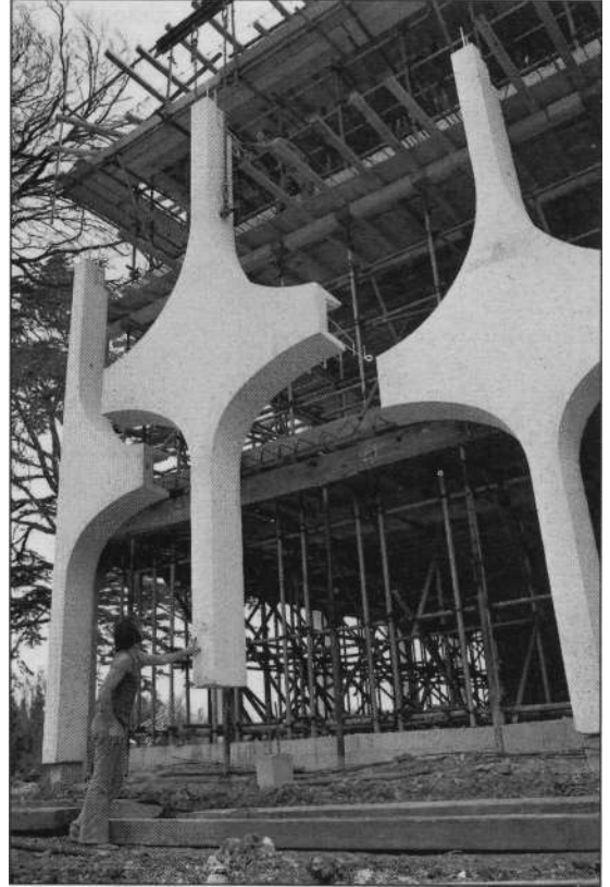
Fig. 4.59 Hybrid in situ /precast structure. In this structure precast concrete perimeter units are used in conjunction with an in situ concrete framework. The superior standard of finish which precasting allows is exploited to allow the units to be exposed on the exterior of the building. [Photo: British Cement Association]
