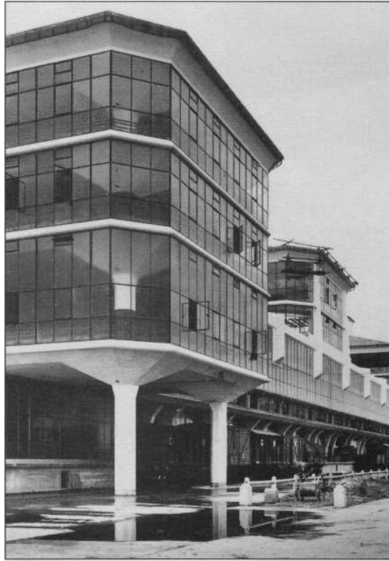
Fig. 4.8 Boots Warehouse, Beeston, England, 1930-32, Owen Williams, architect/structural engineer. The structure here is a two-way spanning flat slab with mushroom-head columns. Its prominence and the transparency of the walls produce a similar tectonic quality to that seen in the Bauhaus (Fig. 4.7) and place the building in the forefront of contemporary architectural development.[Photo: British Architectural Library Photographs Collection]
