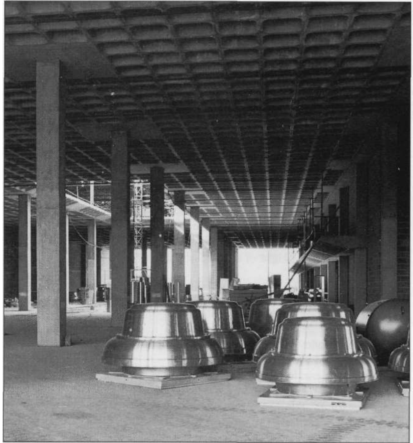
Fig. 4.40 Coffered slab. The coffered slab is a two-way-spanning flat-slab structure (i.e. a slab which is supported directly on columns). The coffers improve the efficiency by removing concrete from the tensile areas where it contributes little to the structural performance [Photo: Pat Hunt].
