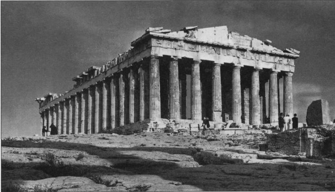
Fig. 5.15 The Parthenon, Athens, 5th Century BCE. This is the most refined example of post-and-beam construction in the Western architectural tradition. The short spans involved are a consequence of the inherent weakness of masonry in tension and therefore in bending. [Copyright: RIBA Photo Library]
