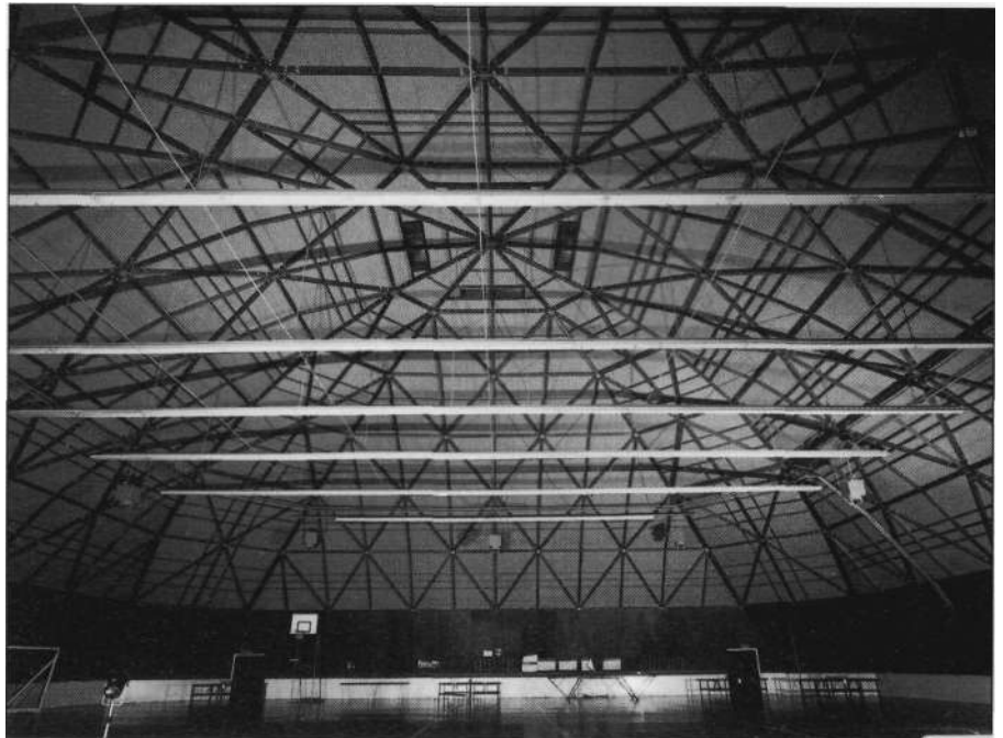
Fig. 6.61 The braced dome configuration allows large interiors to be constructed with a very efficient use of structural material.
