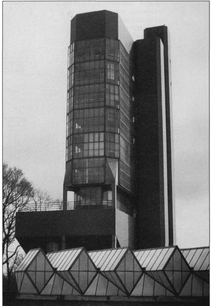
Fig. 4.14 Engineering Building, Leicester University, England, 1965-67. James Stirling, architect, F. J. Samuely & Partners, structural engineers. This building has a reinforced concrete framework structure and demonstrates two of the principal advantages of the material. Its high durability has allowed the structure to be exposed on both the exterior and interior, and thus to contribute to the architectural language being used, and its mouldability has been employed to produce a relatively complex building form (Photo: P. Macdonald).
