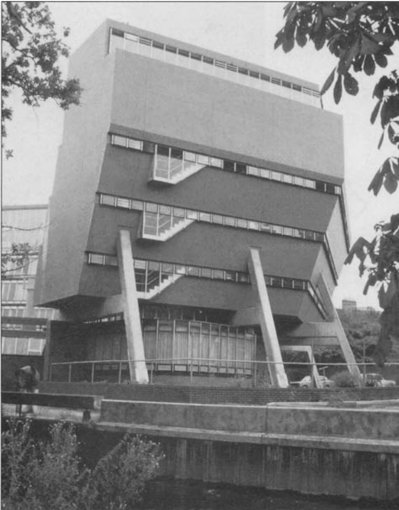
Fig. 2.9 Florey Building, Oxford, England, 1967-71. James Stirling, architect, Felix Samuely & Partners, structural engineers. This building has a fairly complex form which was realised by a relatively straightforward adaptation of a standard reinforced concrete framing system. [Photo: P Macdonald]
