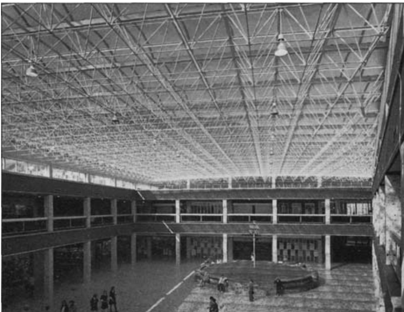
Fig. 3.39 Spacedeck space frame system supported around its perimeter at the Aberfan Centre, Wales. [Photo: Henry Morgan]
