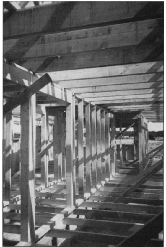
Fig. 1.19 Timber loadbearing-wall structure. Everything here is structural. The wall and floor structures consist of closely spaced timber elements. Temporary bracing elements, which provide stability until non-loadbearing cross-walls are inserted, are also visible. [Photo: A. Macdonald]
