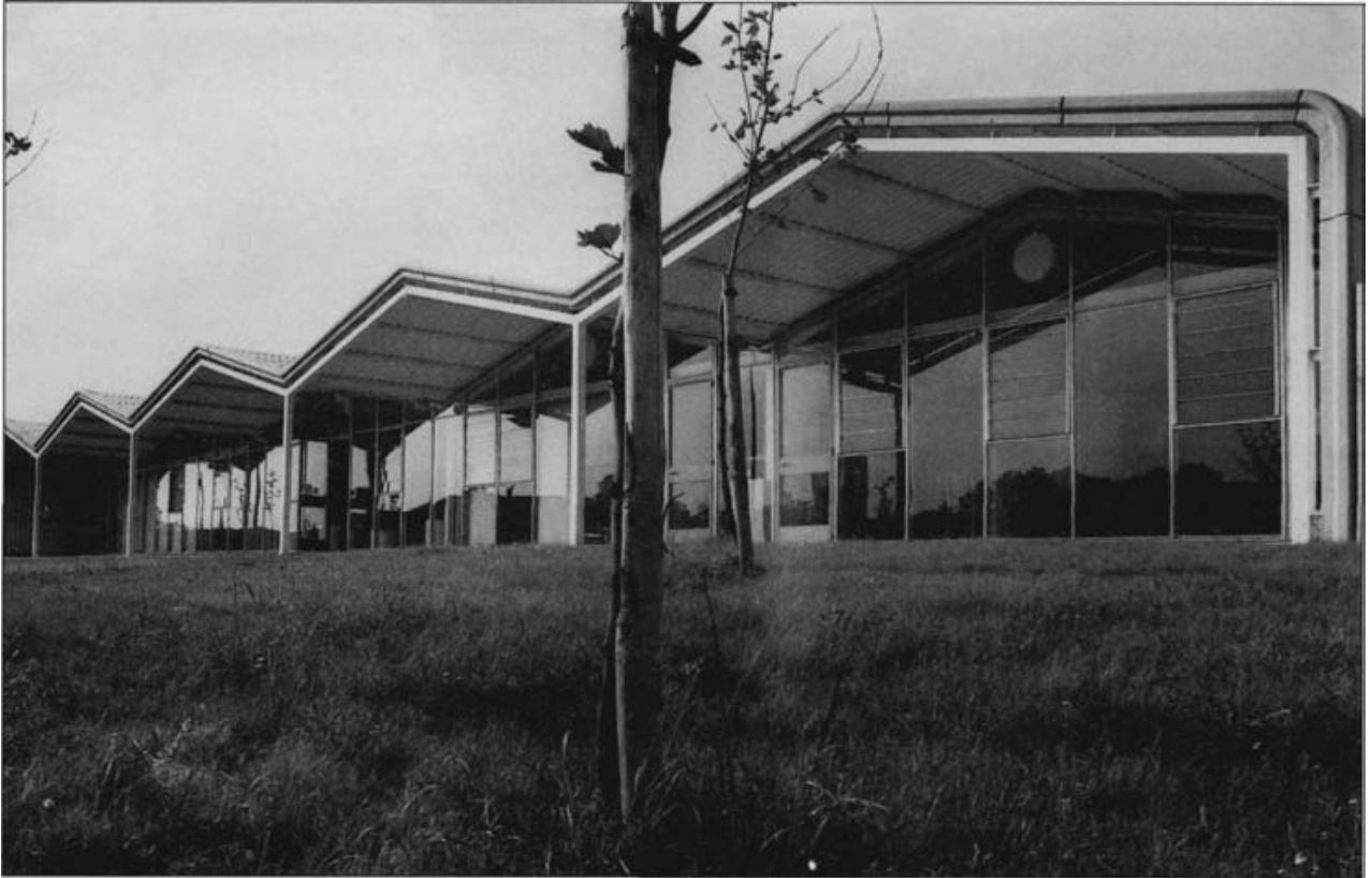
Fig. 1.14 Palmerston Special School, Liverpool, England, 1973-76 (demolished 1989). Foster Associates, architects; Anthony Hunt Associates, structural engineers. Semi-form-active portal frames of steel hollow-section are used here as the primary structural elements in a multi-bay arrangement with relatively short spans. The moderately high efficiency of this type of structure has permitted very slender elements to be adopted. [Photo: John Donat]
