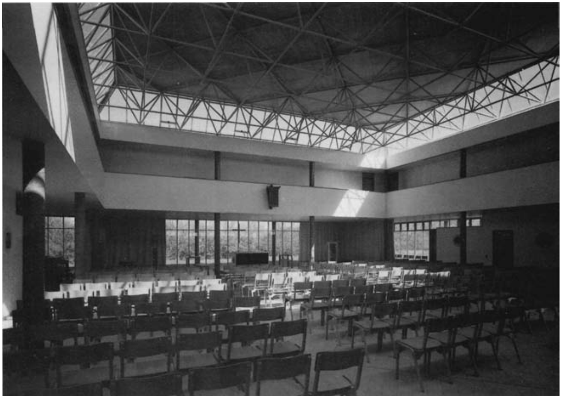
Fig. 3.40 (a) Basic components of the Mero space frame. This highly versatile system allows great freedom to the building designer because the lengths of the elements are not predetermined. It is possible to use this system to create a wide variety of structural forms including domes and vaults as well as flat space decks, (b) Church, Milton Keynes, England, with Mero spacedeck roof. [Photo BICC]
