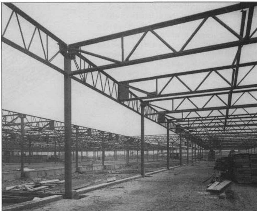
Fig. 3.27 Castellated beams are arranged here in one of the standard configurations for single-storey steel frameworks. [Photo: Pat Hunt]
