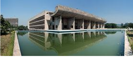
Le Corbusier, Assembly building, Chandigarh, India
