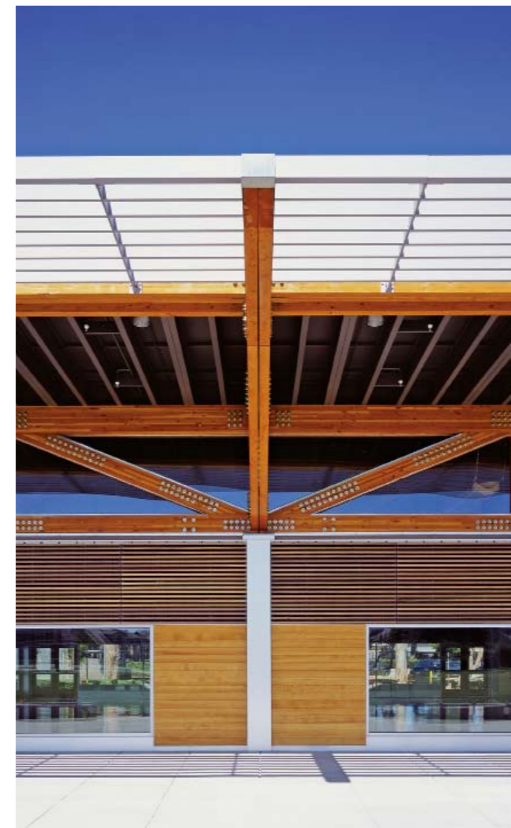
Detailed exterior cedar and glass façade of multi-purpose pavilion on west, south and east sides
