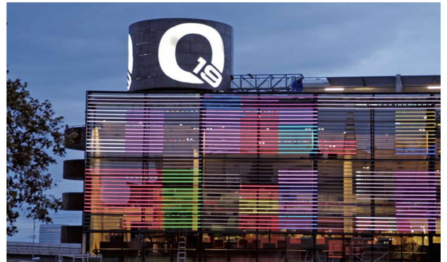
Façade – LED façade, entrance
