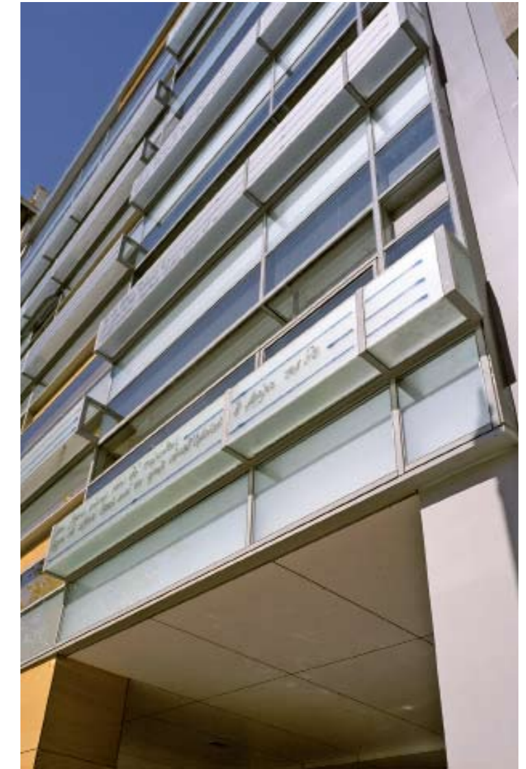
Details of façade
