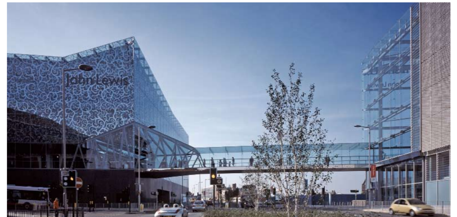
Façade with bridge
