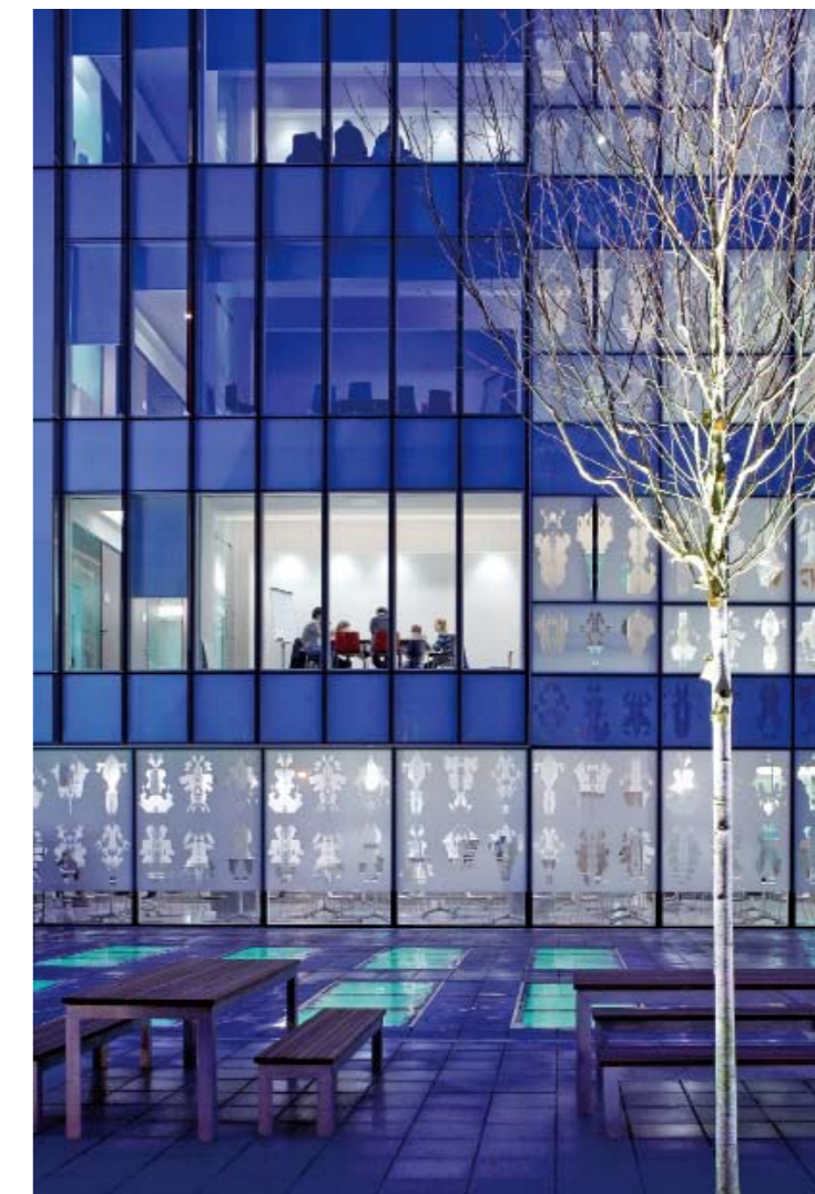
The exterior glass façade around the entrance courtyard, with Nicky Hirst's artwork The Glass Menagerie .
