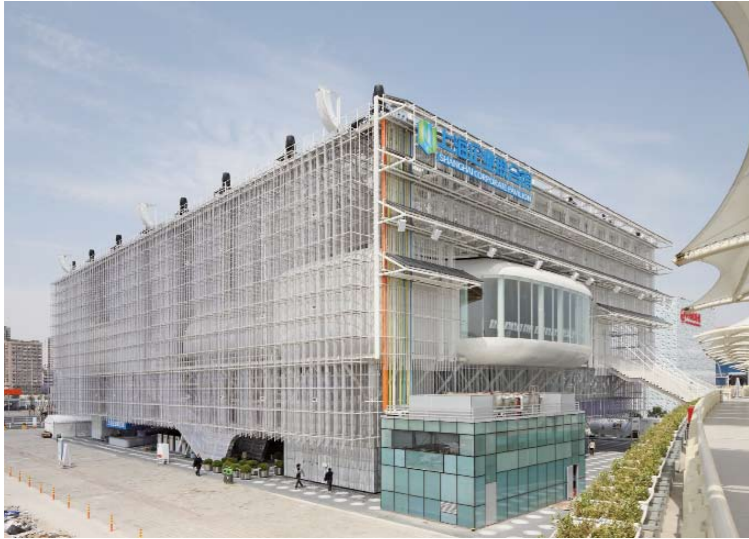
View from southwest
