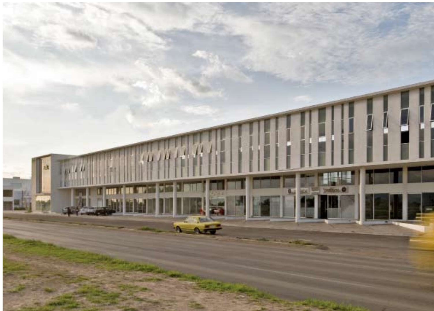
It is an almost 100-meter-long building, with a series of vertical strips used for ventilation by tip-up windows
