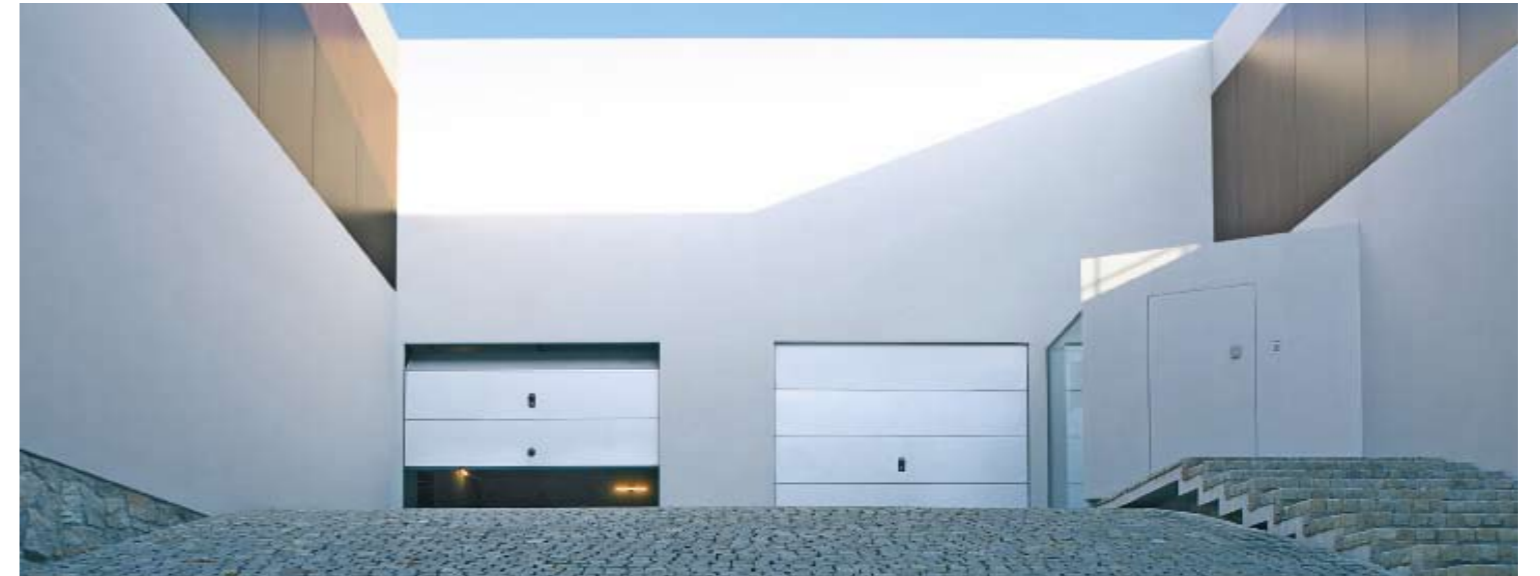
A view of the atrium
