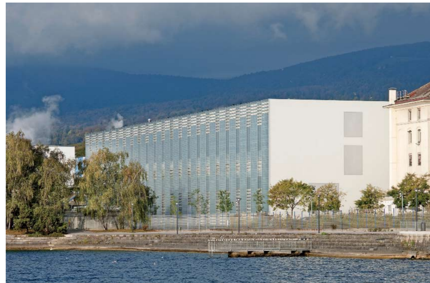
South Façade, took from the Neuchâtel Lake
