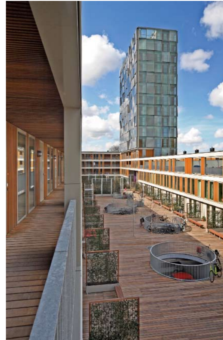
Courtyard on the roof
