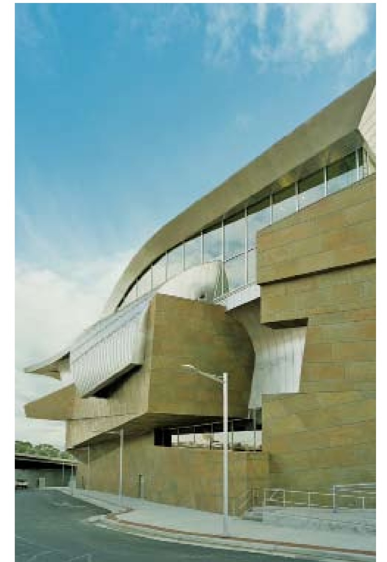
Exterior view from Norfolk Avenue
