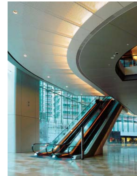
Escalators at ground floor
