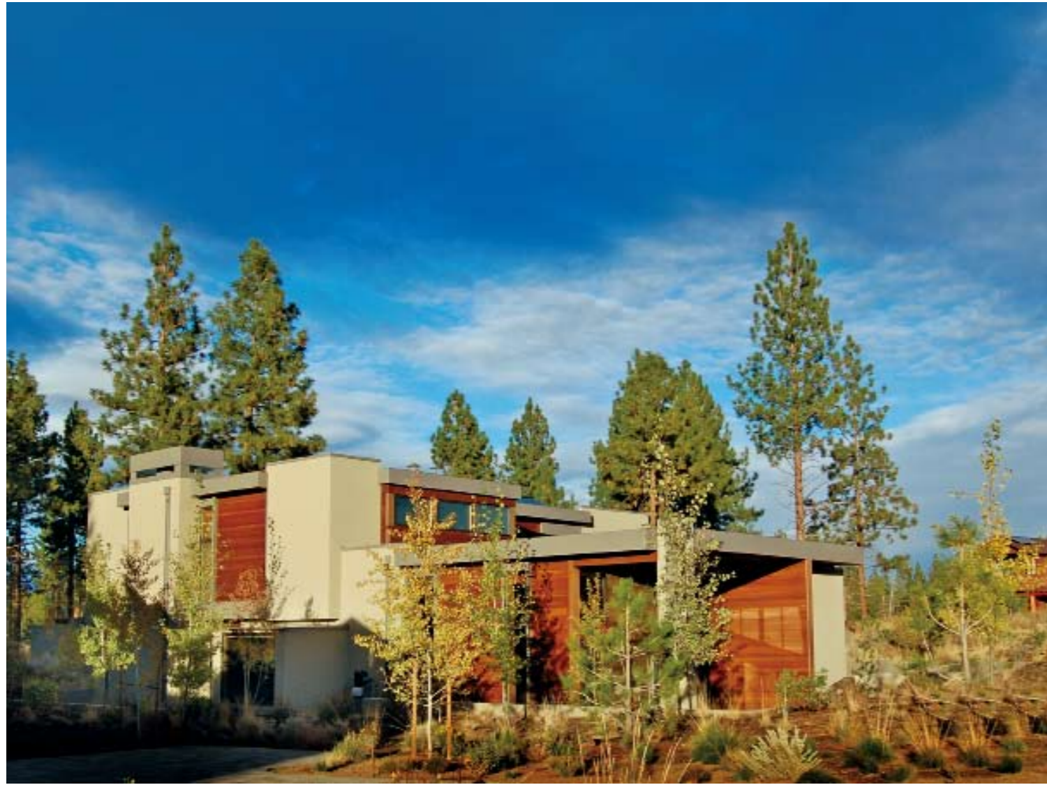
Building in the evening
