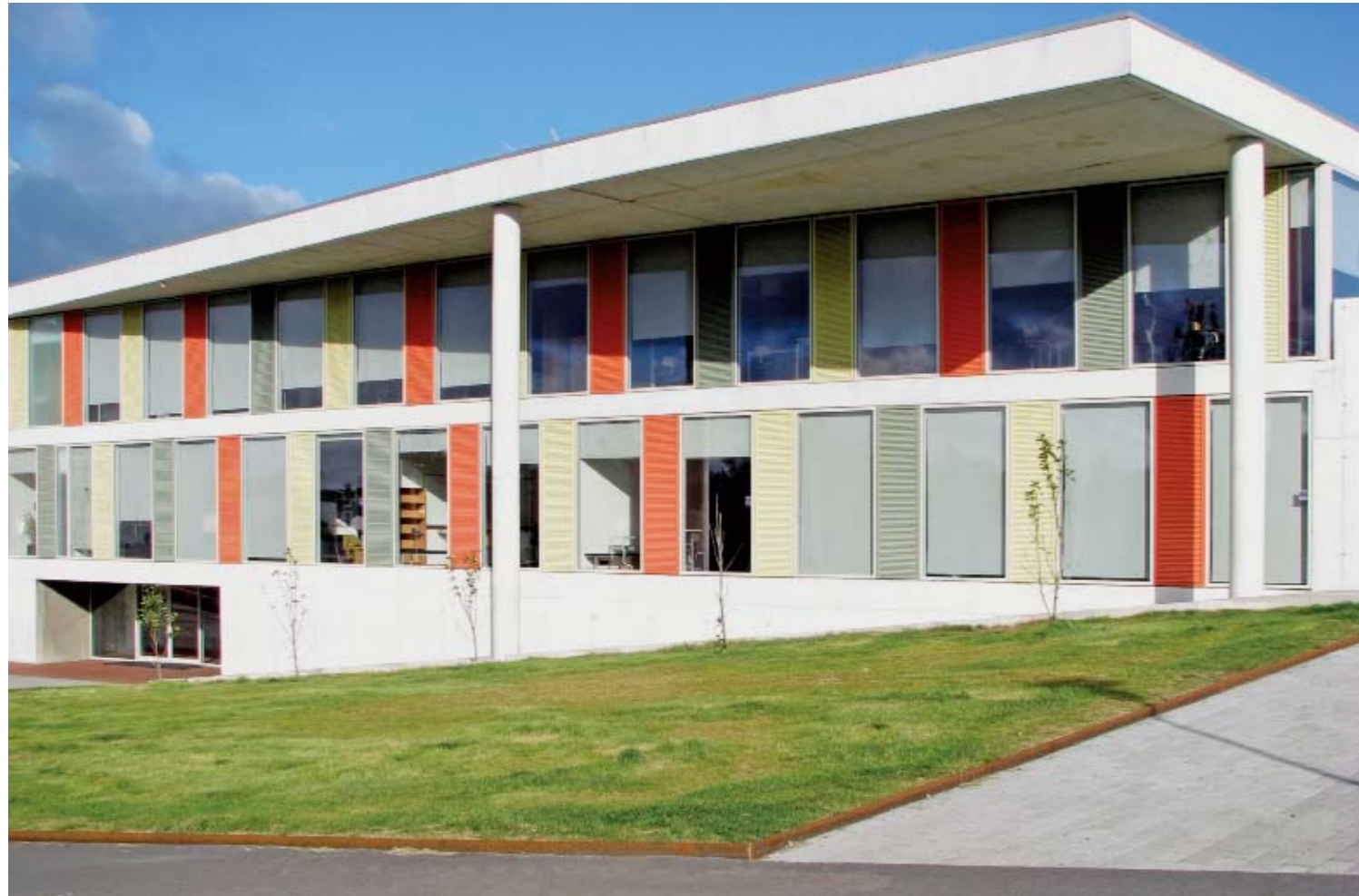
Stepped ramp and canopy on south side
