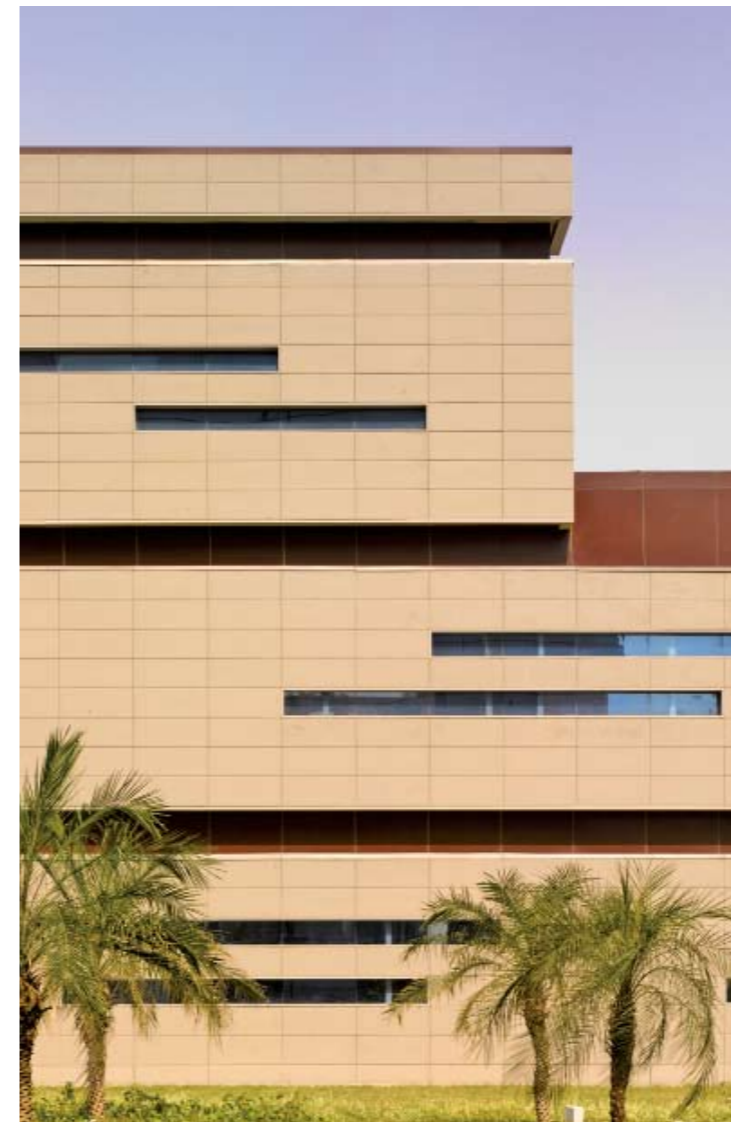
Shaded outer façade with small slit windows
