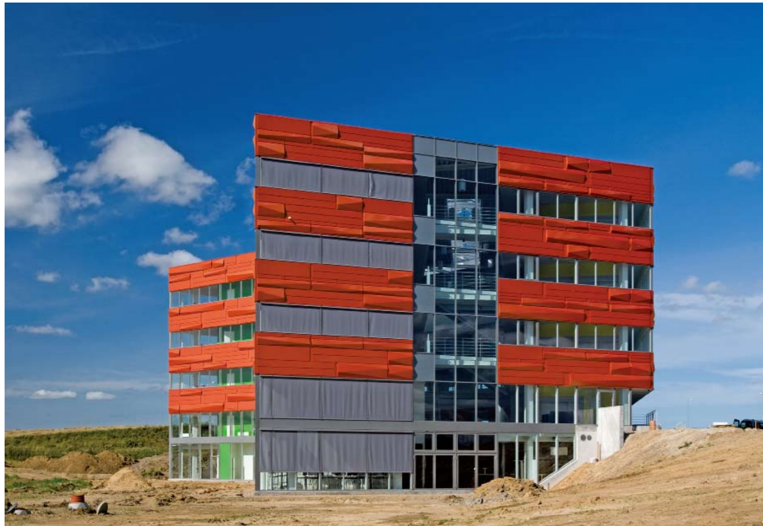
View from the south
