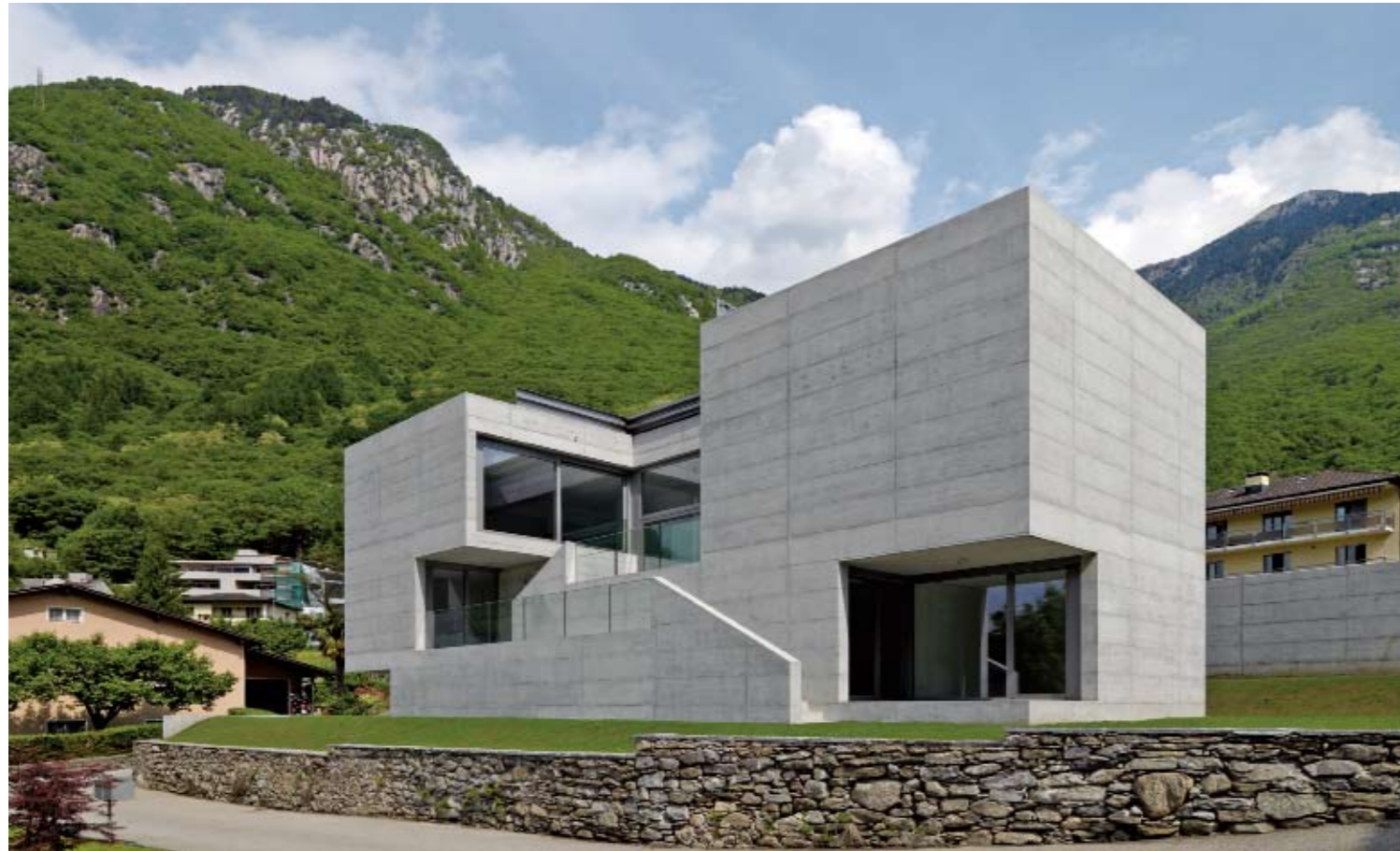
External view of the house in its Alpine context from the southeast
