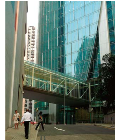
Footbridge to OIE
