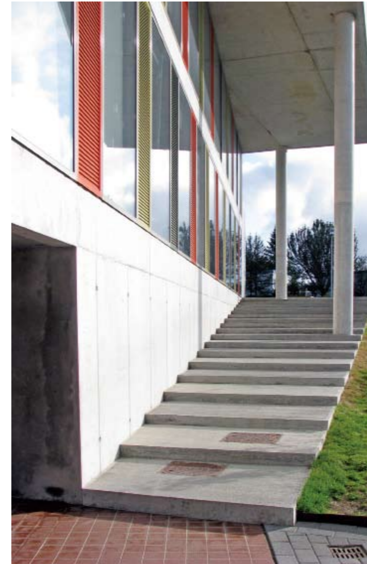
Stepped ramp and canopy on south side
