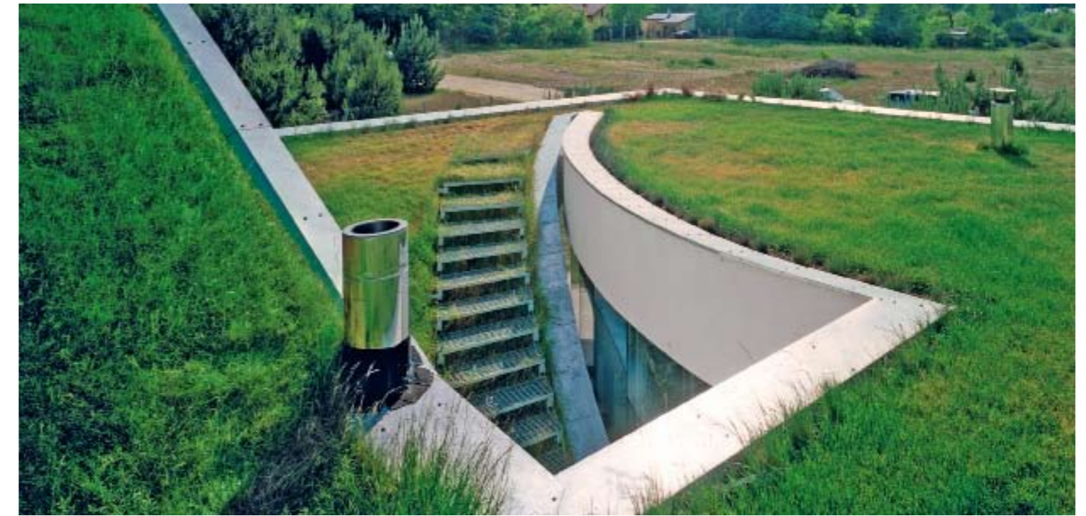
The stairs leading to the roof with one mesh across which grows the grass
